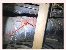
Damaged ductwork insulation should be repaired as needed.
