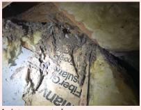
Moisture ant damage was noted in the framing at the west side - I believe this is where the concrete walkway meets the building. No live ants were found.
