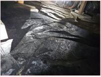
Active plumbing leaks were noted below the main bath tub
