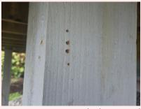
Carpenter ant exit holes noted in deck framing - risks concealed damage. See east deck posts
