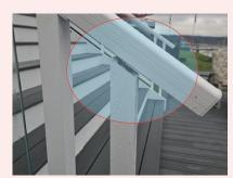
The bottom posts for the metal guardrail are not secured properly to the handrail
