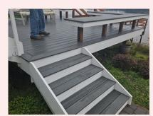
The back deck stairs are missing a proper graspable handrail
