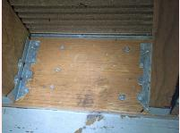
The newer east deck has a nice ledger that has been bolted to the building
