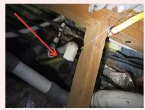
Condensate lines are draining into the crawl space. This should be repaired - all condensate should terminate to the exterior
