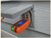
The GFCI protected receptacle on the exterior south side did not trip when tested
