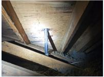
Localized darkening was noted in the attic - particularly around exposed nail heads and at dead air spaces.
