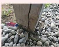
Wood decay was noted at the base of one of the non-treated east deck posts
