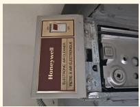
The furnace filter was shut off at the time of inspection indicating it is not operating
