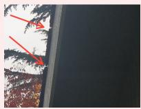
Damaged rake edge shingles noted
