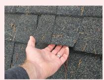
Shingles are getting older and not bonding as well. They will be increasingly vulnerable to wind damage.
