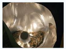
Older can lights were noted that likely leak air into the attic
