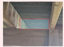
Blocking is missing at the joist to beam connection - these are recommended for sheer strength. East Deck
