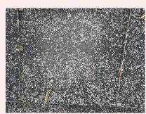
Moderate to heavy granule loss on the shingles
