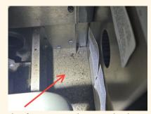
The furnace is dirty at the base of the burner assembly
