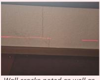
Wall cracks noted as well as roughly 1 inch of settlement
