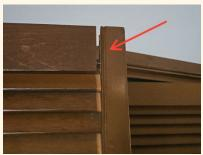
The bifold doors to the water heater closet in the office are damaged
