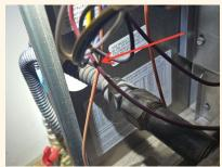
The gas supply connector is run through the gas furnace cabinet - this is not allowed
