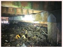
The 4x4 for the west landing beam is sagging.
