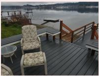
The lower deck here would be required to have a guardrail where there are bench seats.
