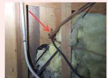
Holes in the sub-floor should be air-sealed prior to re-insulating.
