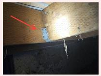
Hangers are not sized correctly for the joists. Hangers should be at least 60% the depth of the joists. West Landing
