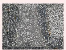
Fairly heavy granule loss noted on the roofing shingles
