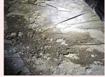
The clear plastic vapor barrier is damaged, incomplete and inadequate
