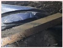
Wood debris should be removed from the crawl space - this is conducive to wood destroying organisms
