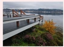
The guard has a bench built into it that is unsafe for children and does not comply with required guardrail standards.
