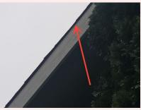
The roofing shingles do not adequately overhang the fascia at rake ends. These should hang off at least 1 inch.
