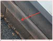
Some of the holes to secure the skylights are missing fasteners
