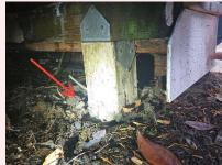
Eliminate post to soil contact to prevent wood decay in the base of deck posts. West landing
