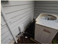
No electric receptacle is noted for servicing the heat pump
