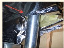
The foil paper in the attic appears to be too close to the furnace flue - be sure there are adequate clearances here.
