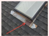
Mild corrosion noted on the skylight flashings
